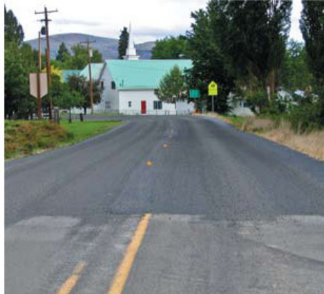
If you see a change in the color or texture of the surface ahead, it's smart to conserve traction until you figure out what the appearance change really means. Actually, this is gooey road oil covered with a deep layer of loose gravel. Photos by David L. Hough.
